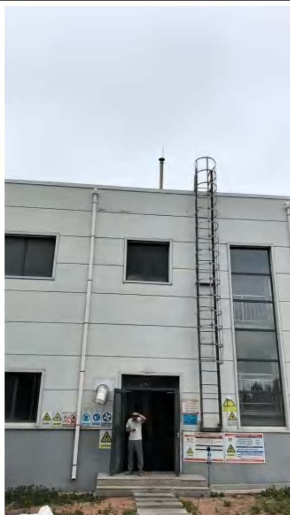
拆炉尾气排气筒 DA003
