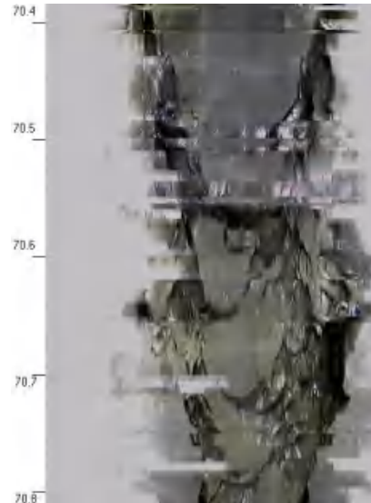
图8.3-12 70.4~70.8/57.67m深处垂向裂隙
