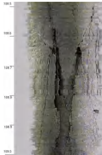
图8.3-13 108.5~109/88.88m深处垂向裂隙
