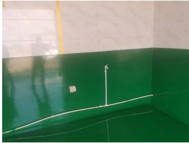
裙角涂刷环氧树脂漆
